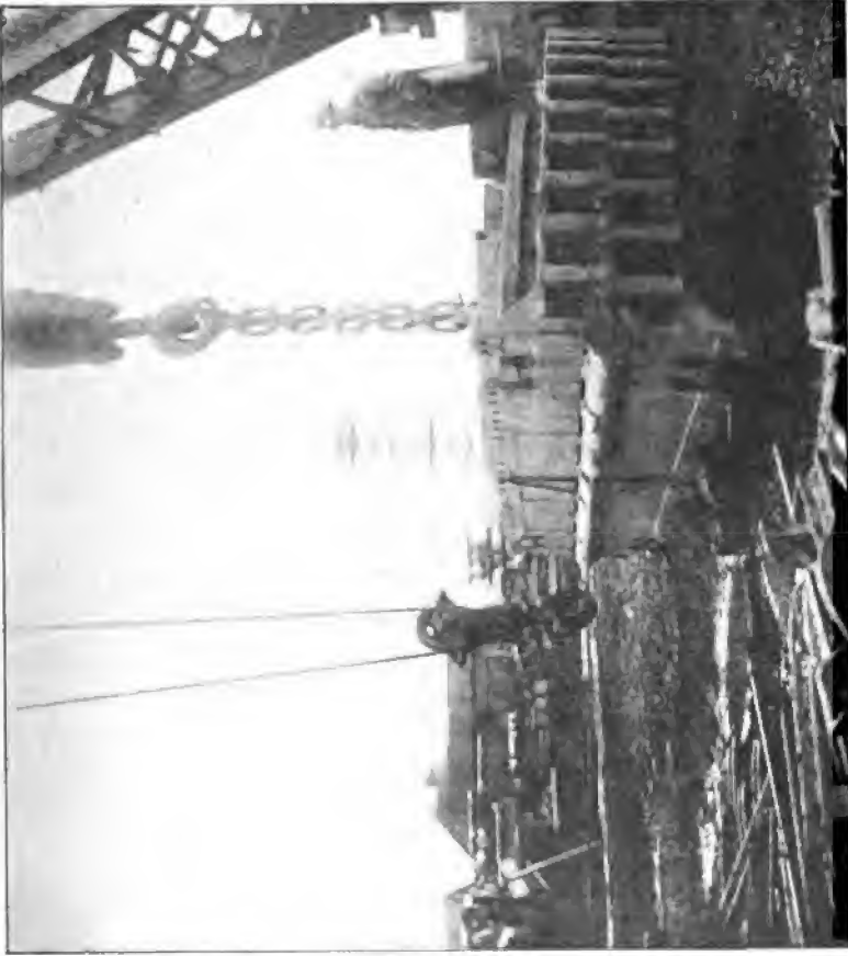
BASE RING OF THE 14-INCH, 45-CALIBER AMERICAN GUN MOUNT, MODEL "E" (FIRST STEP OF INSTALLATION).
